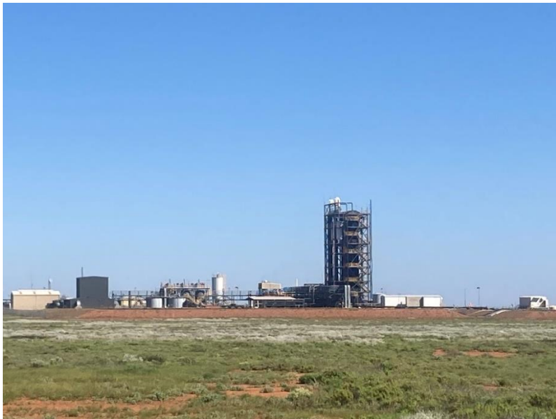
Figure 4: Honeymoon plant, including soon to be replaced solvent extraction columns
