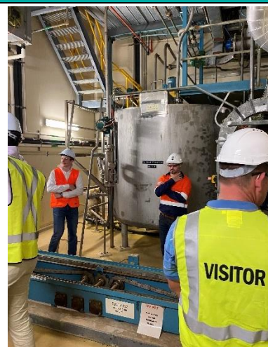
Figure 6 – Uranium packing facility
