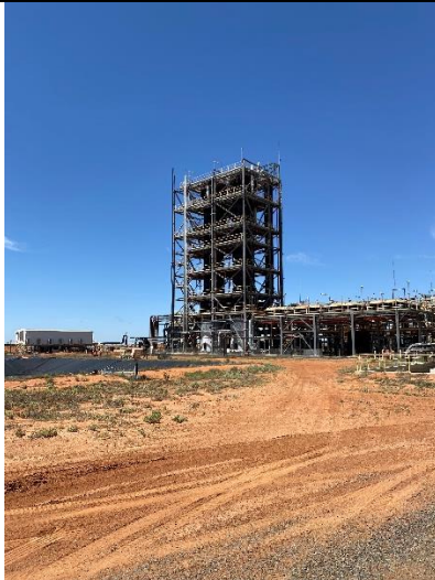
Figure 3 – Existing SX columns to be replaced with IX
