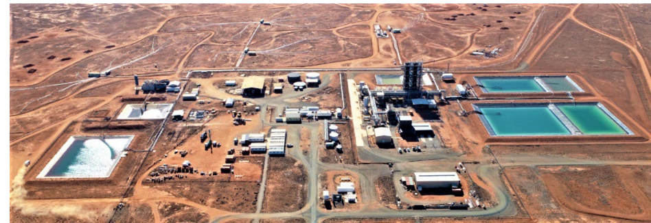
Honeymoon Processing Plant and Wellfields, South Australia
