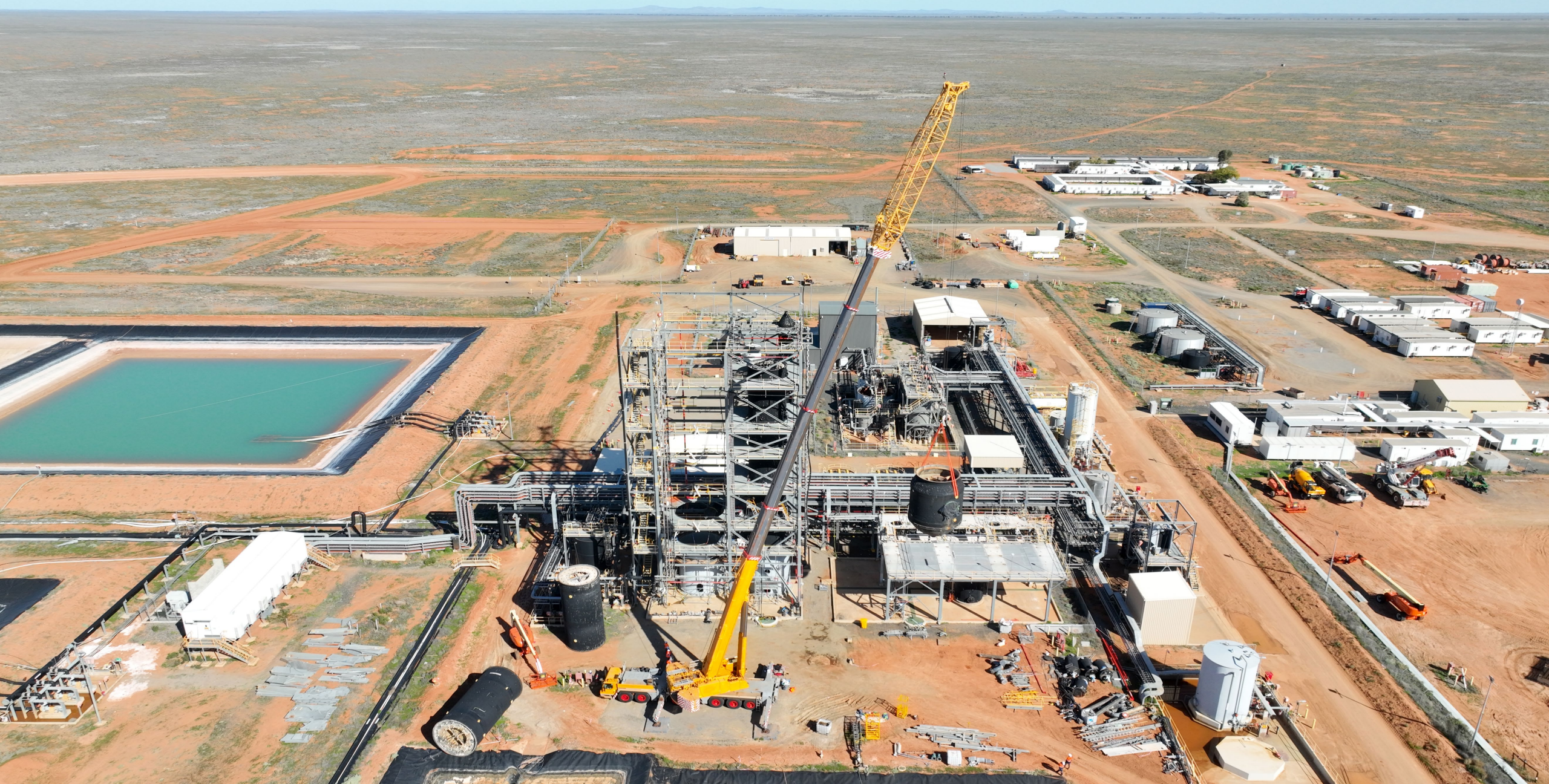
Boss owned 400T crane removing redundant Solvent Extraction pulse columns
