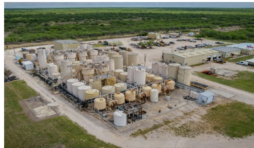
Alta Mesa Processing Facility
