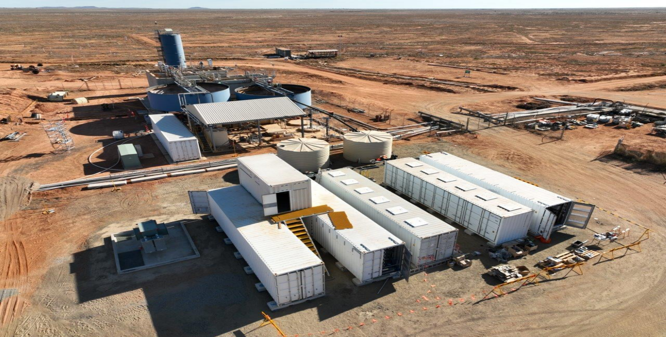
RO and Water Treatment Plant
