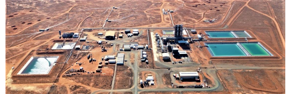
Honeymoon Processing Plant and Wellfields, South Australia
