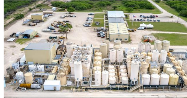
Alta Mesa Central Processing Plant, Texas, USA
