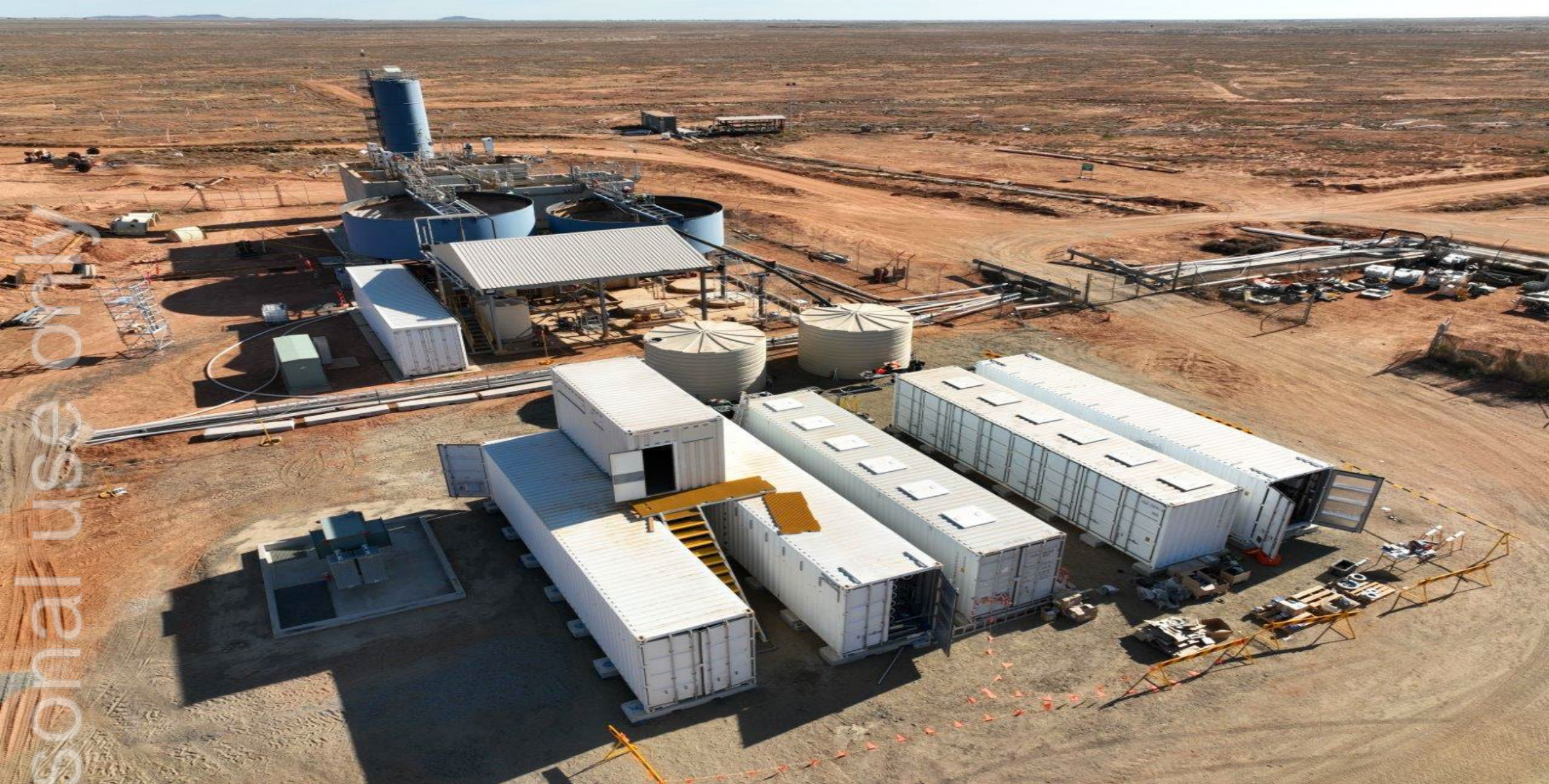
RO and Water Treatment Plant
